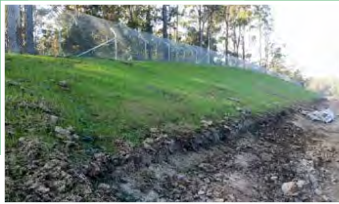
Bonded fibre matrix application germination following rainfall.
