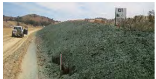
Application of a Bonded Fibre Matrix. The application itself only included minimal fertilisers and seed in accordance with a standard RMS R178 specification.
