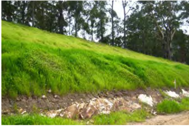
Results of Ameliorated Application to rocky areas with limited topsoil on the Hunter Expressway
