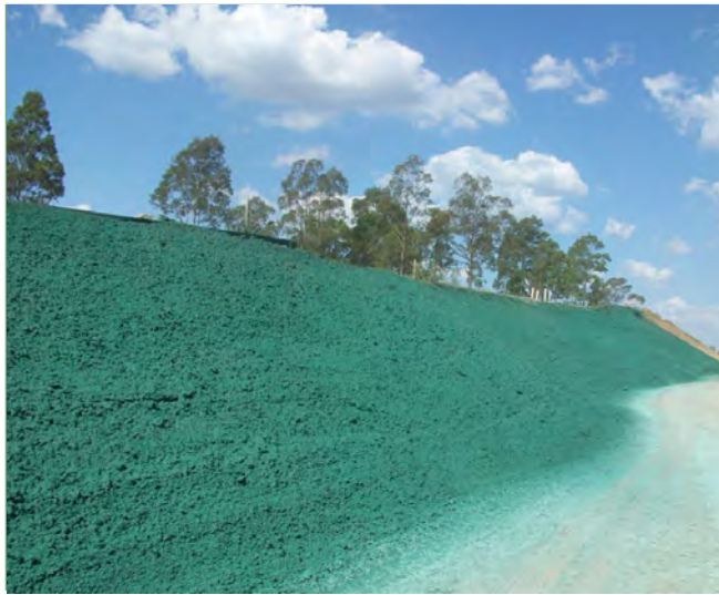
Application of Ameliorated Hydromulch
