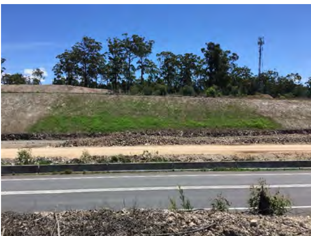
Figure 15- Cut 5 NB 10th Nov 2015 - Ameliorated Mix over failed Specification Mix - Topsoil scarified on lower section of batter only with improved germination.
