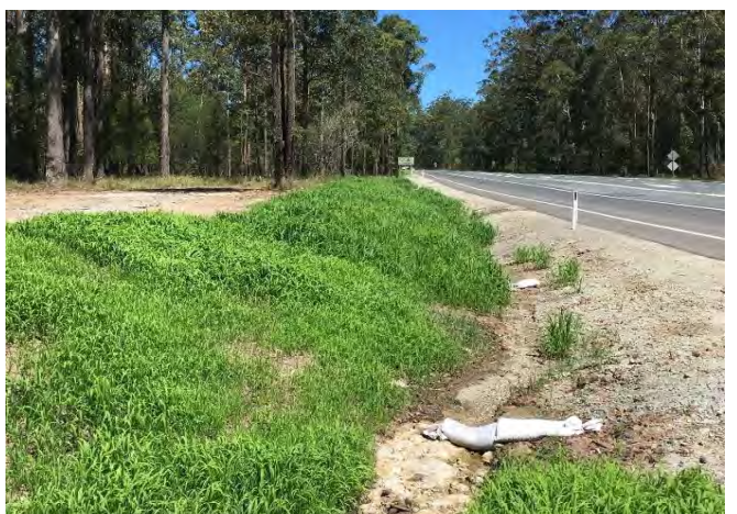
Figure 17 - Bill Hill Road Intersection 10th Nov 2015 after 173.3 mm Rainfall since 29th Sept 2015 - Dense healthy grass on loose topsoil surface
