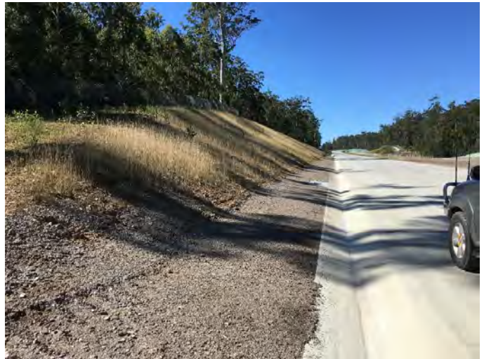
Figure 3 - Standard Hydromulch typical batter where initial cover crop germination has hayed off due to lack of long term nutrition.
