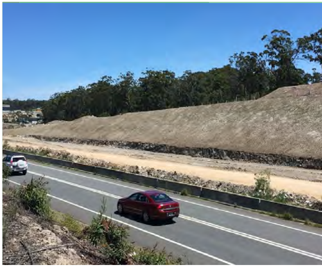
Figure 1 - Cut 5 NB Nov 2015, Failed Standard Specification Mix
