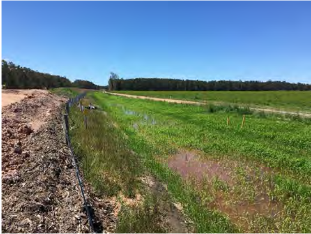
Figure 14 - Fill 13 SB Drain 10th Nov 2015 after 173.3 mm Rainfall since 29th Sept 2015 - Dense healthy grass on loose topsoil surface
