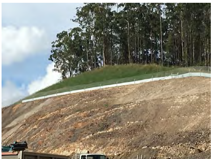
Figure 5 - Cut 19 NB Ameliorated Mix Application, Upper Batter 10th Oct 2015
