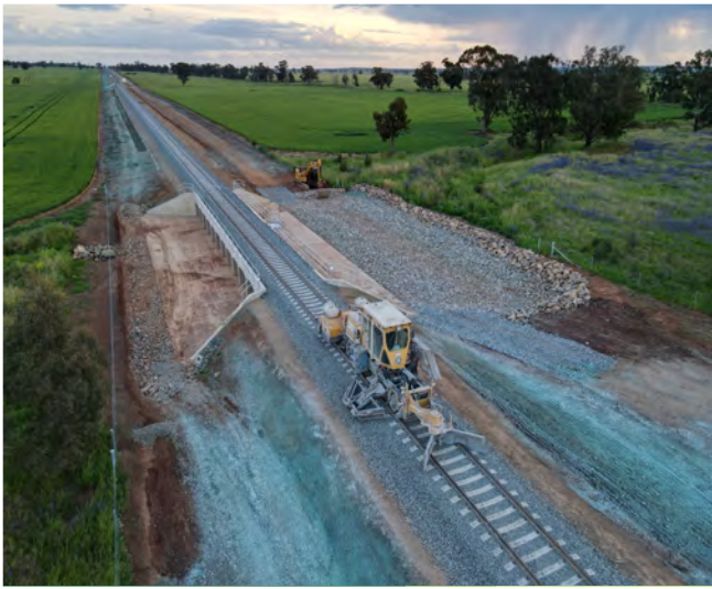
Application of Ameliorated Hydromulch
