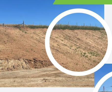
On this area we applied a Standard Hydromulch application, which failed because there was not enough nutrients in the soil to stabilise the seedbed and allow for germination. As you can see, the batter did not wash away and remained on the surface.
